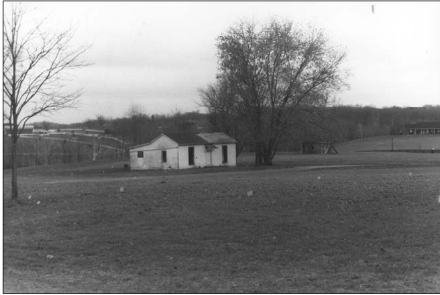
Figure 4. Tenant House Just Before Demolition in 1998.
