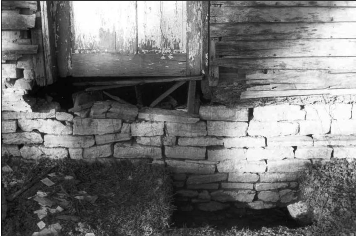
Figure 11. Foundation of Two-Room Frame Structure.
