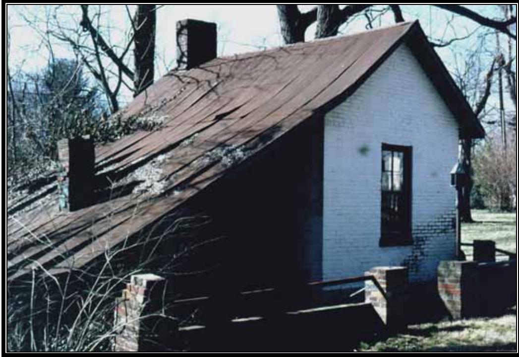
Figure 5. Multipurpose Building with Washhouse at the John Herr House.
